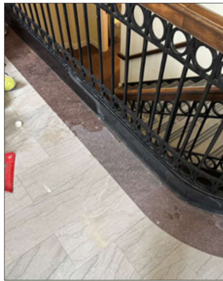
Slapwax on the Belgian Black baseboards. Right: Restoring the stairs involved some serious (and tedious) handwork.
