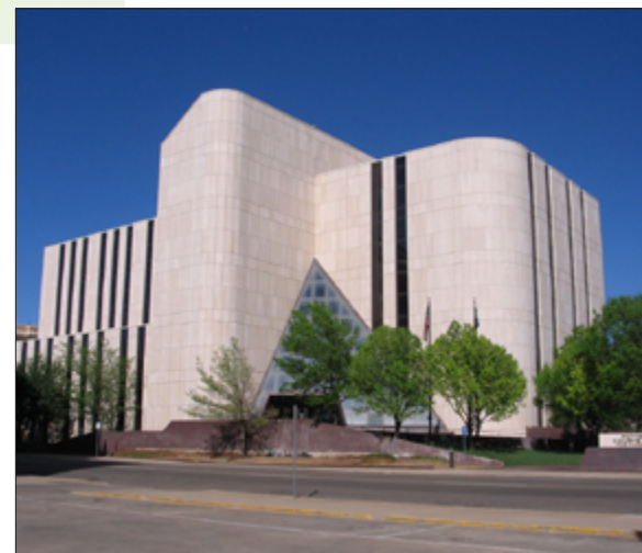
The Potter County Court Building, Amarillo, Texas features a façade of Continental Buff vein-cut travertine.
