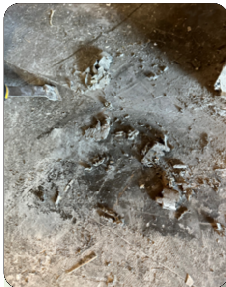
Getting down to the concrete involved lots of scraping with razor blades. Just look at this mess!
