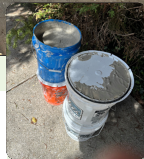
Buckets of slurry, from grinding wet, had to be carried offsite for disposal.
