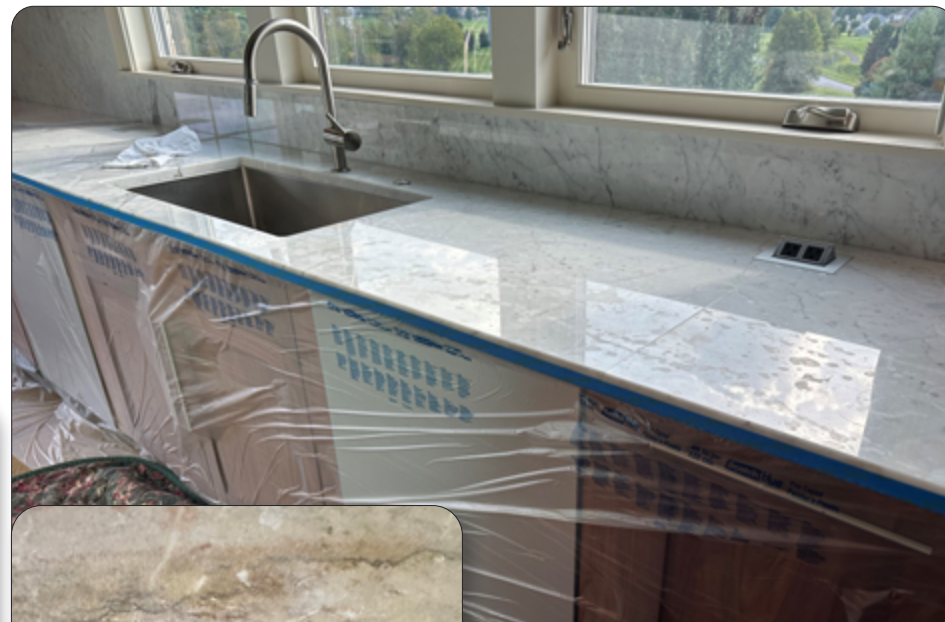
Marble countertop with etching all over the surface.
