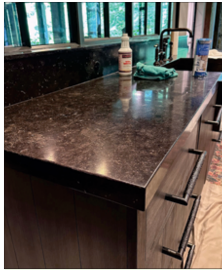
Finished restoration on the higher honed darker material.
