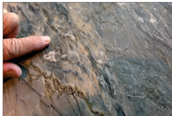
The scratching is so deep on this limestone countertop that you can catch it with your fingernail.
