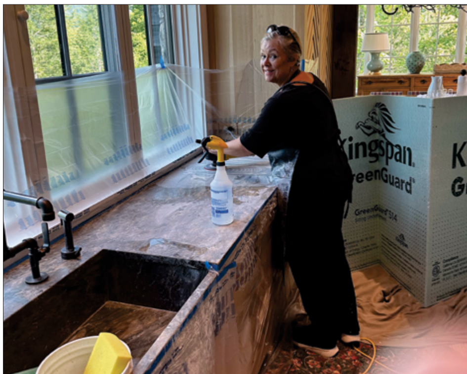
Julie running a 200 grit ELF5 Flexible Metal-Bond 120 grit on the heavily scratched and etched areas.
