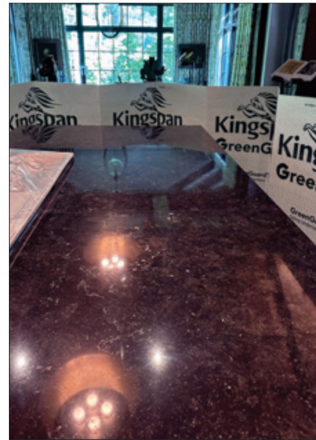
The final high hone look on the island. Notice the Tape & Drape, masking, and portable wall for protecting the surrounding surfaces.
