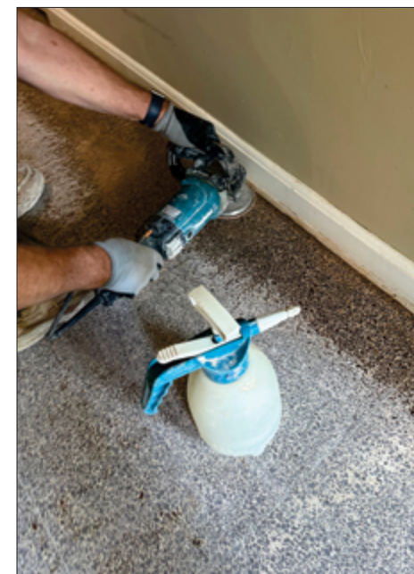
Cutting in the borders with a Makita and ELF5 40 grit flexible metal bond.
