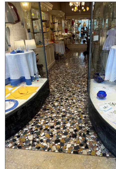
A quilt marble floor in a shop in Venice. Most of the stone flooring we noticed in Italy was honed.
