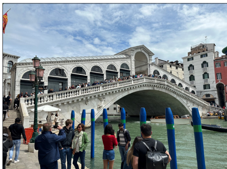
The famous covered Rialto Bridge, In Venice – an amazing marble structure.
