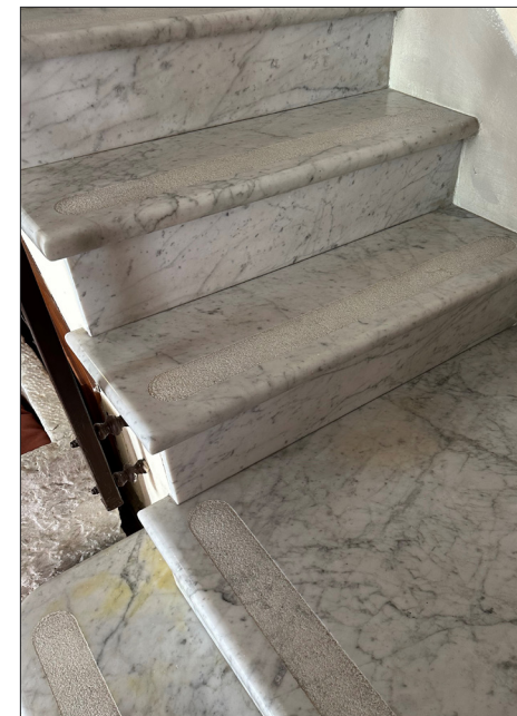
Honed marble steps in a restaurant. Notice the integral traction treads, which are likely from somewhat newer technology!
