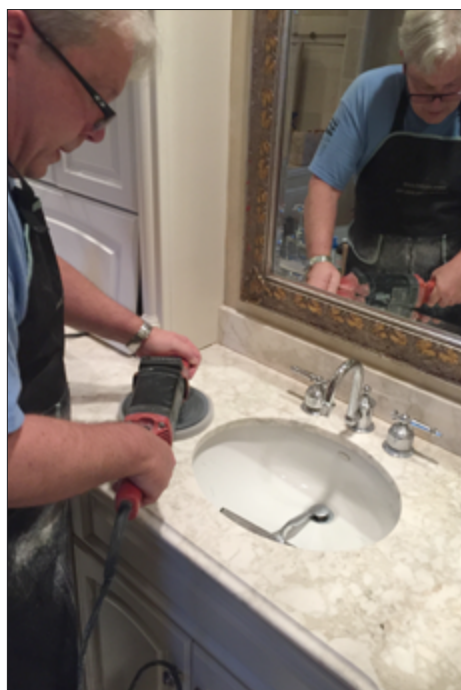
Adding finishing touches on a marble vanity using an older Flex 302.
