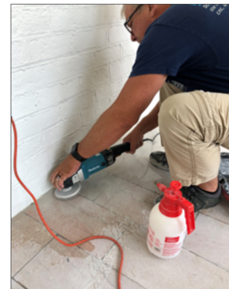
Lippage work on Tennessee Pink marble using an ELF Flexible Metal mounted on a Makita grinder.
