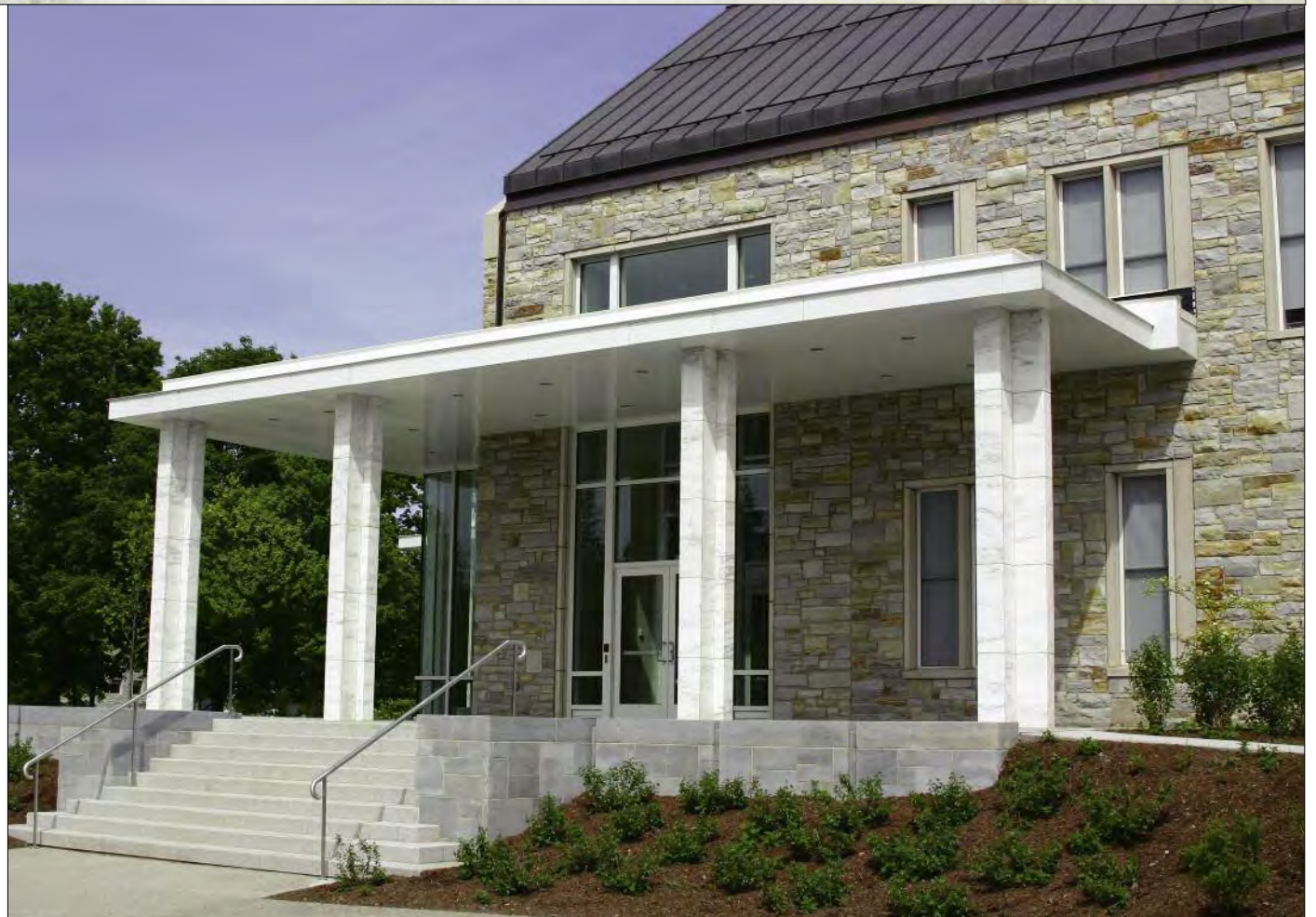
Front entrance to the Shepley Pavillion Reading Room features Danby-Marble-clad pillars and "split-face Middlebury College blend." Middlebury College in Vermont is noted for its stone buildings and use of stone native to the granite and marble-rich Barre area.
